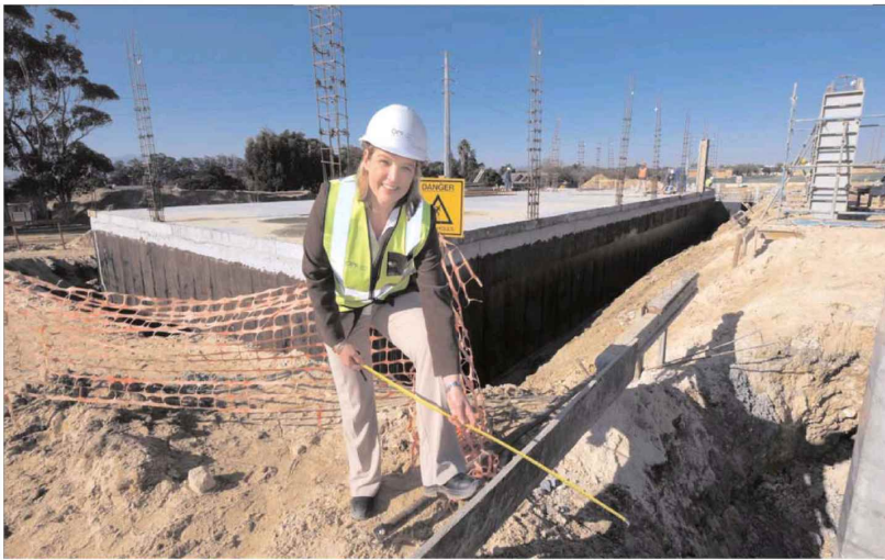
MEASURING UP: Quantity surveyor Alison Ahmad struts her stuff at a construction site in Kraaifontein, where a new showroom for a car dealership is being built. Picture: IAN LANDSBERG
